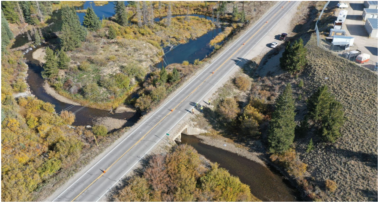
Picture 1 – Bridge G-12-C General Location
